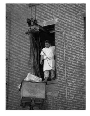
**Figure 1.11** Pulleys make it possible to lift large, heavy loads.
